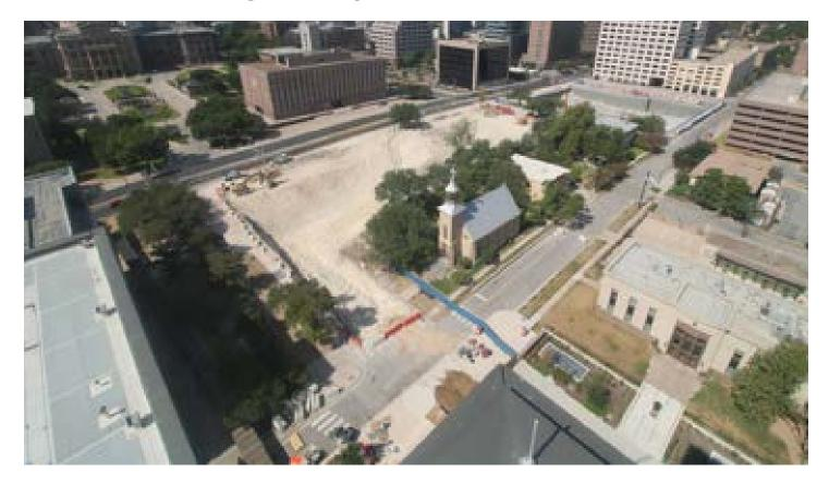
Work is now underway on all three sites of the Phase II project. Ongoing work at the 1501 Lavaca site includes mass excavation and material removal with shotcrete and rock anchor installation. Excavation will continue through the end of the year.
