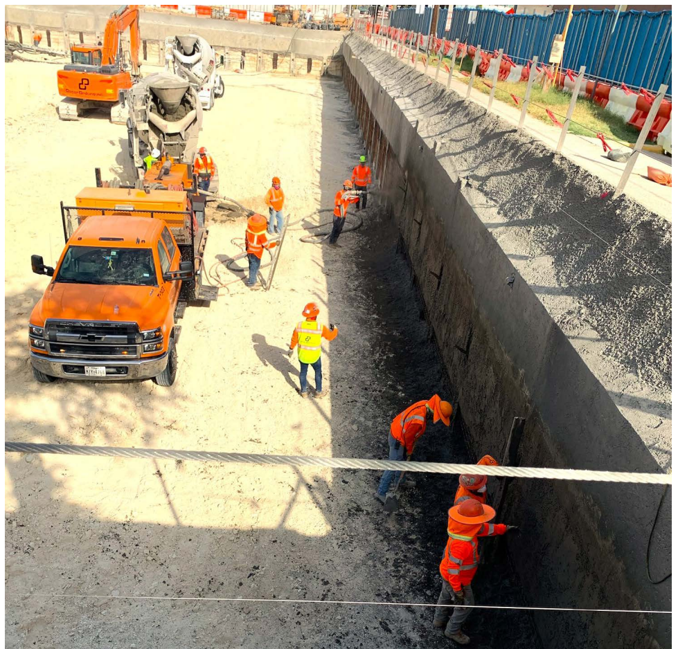
The team applies shotcrete to the wall face.
