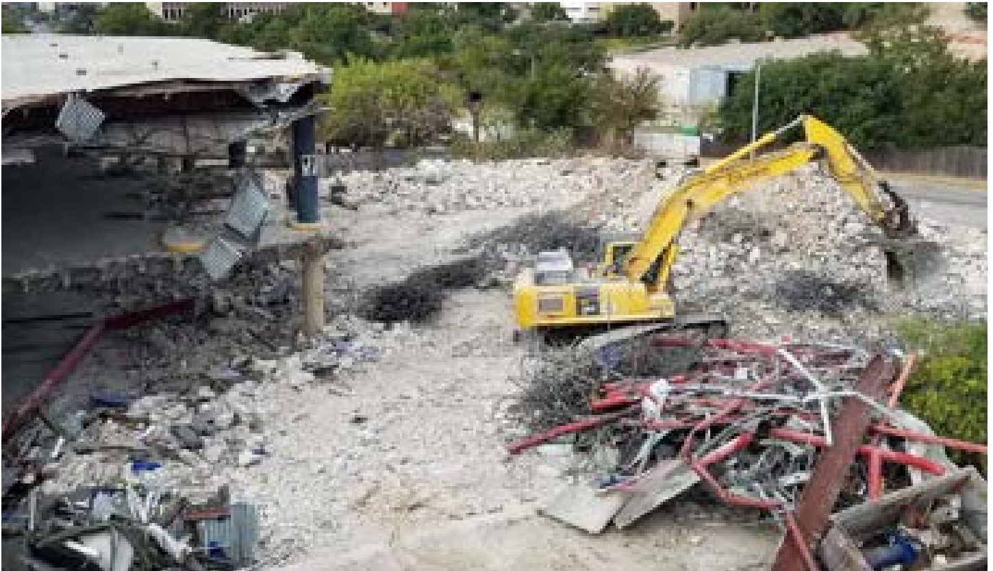
JR RAMON separates construction waste during demolition.
